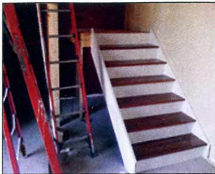
Left: A stair stringer is assembled using EZ Stairs' brackets in the Palm Harbor Homes factory. The brackets are screw attached and then swiveled into place, making stringer set up fast and easy for both risers and treads. This system provides for stair construction either in the plant (center photo) or at the home site. At right a Palm Harbor model featuring stairs built with the EZ Stairs system.
